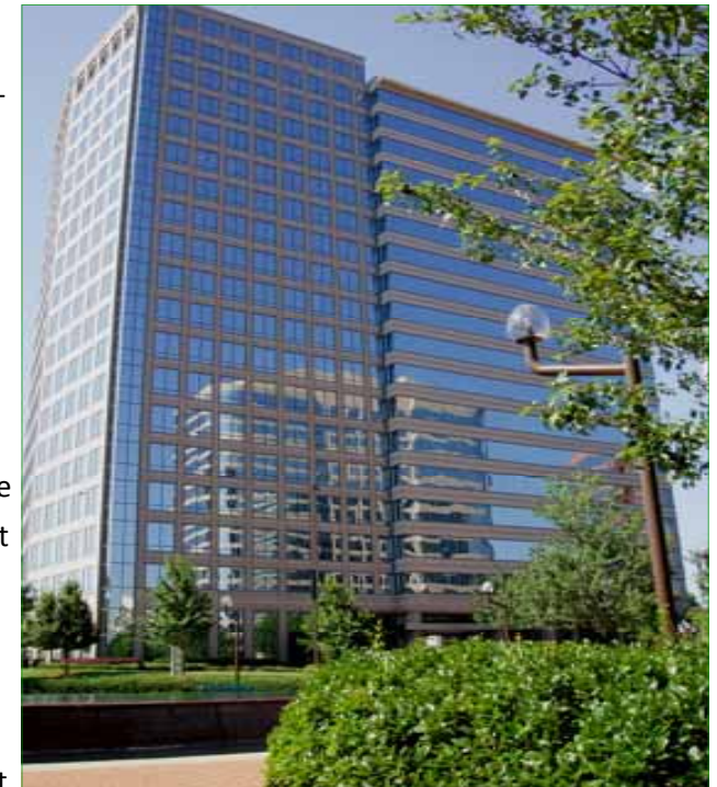
Photo: Office building in Cumberland.
